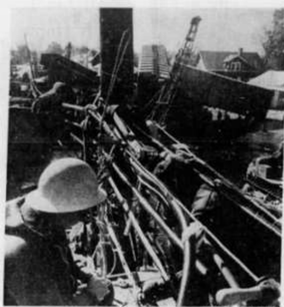
A REPAIRMAN WORKS to restore Crestwood telephone service, which was cut when a freight train derailed near the business district and damaged four cables. The repairs were completed by late afternoon.
